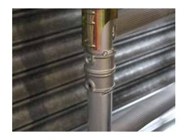
5. Place a brace frame between the 2 frames on the opposite side of the base brace frame with the hooks facing outwards positioned above the bottom rung and 3rd rung of the 2nd 1m frame just above the frame clips (see photo)
