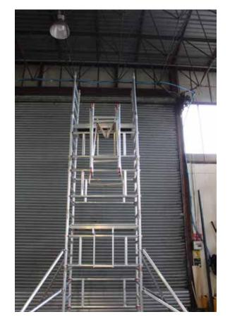
18. Now climb up to and through the trapdoor of the platform until you can sit on the platform with your feet on the rungs below (3T method) While sat on the platform take one of the brace frames from the assembly bracket and position on the opposite side with the hooks above the second rung and top rung of the 5th 1m frame.
