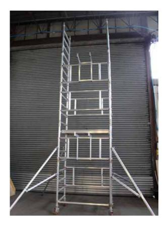
15. You will now need to return to the bottom of the tower and place the remaining 2 brace frames, folding toe board and second platform onto the lower assembly bracket. (see photo)
