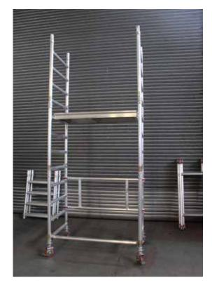
7. Attach the 1st assembly bracket to the top bar of the brace frame, place three of the unused brace frames onto the bracket (see photo)
